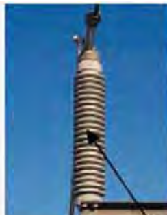
Ceramic Stress Tracking - Corona
