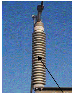
Ceramic Stress Tracking - Corona
